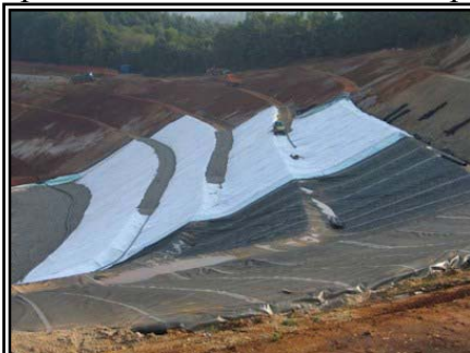
Figure 3. Installation of combined geosynthetic materials
