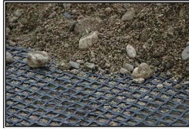
Figure 1. Setting up a geogrid
